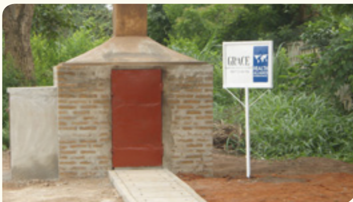
Incinerator funded by GRACE and supported by MOH.
